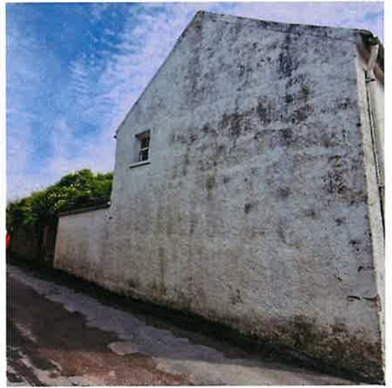
Image C & D above from 28 th August 2024 during Derelict Site Report Inspection: Signs of roof damage and side elevation paintwork / plasterwork dirty and the rear open space overgrown of the property.
