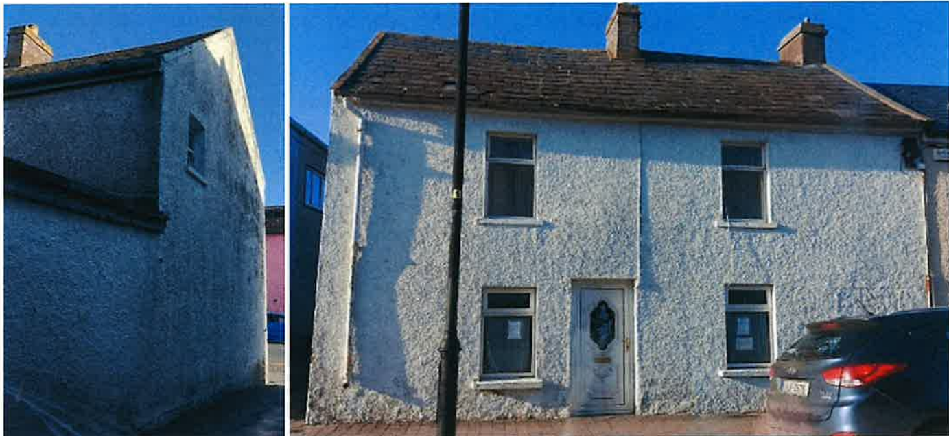
Images K & L above from 28 th March 2025, side elevation and front elevation with damaged roof, gutter, downpipe and flaking paintwork. No change in the condition of the property at Main St., Ardmore.
