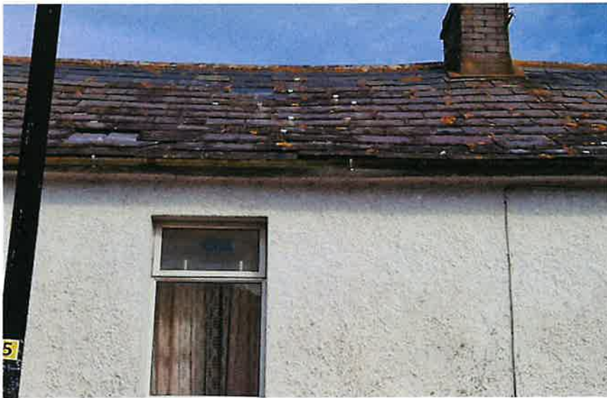
Image C & D above from 28 th August 2024 during Derelict Site Report Inspection: Signs of roof damage and side elevation paintwork / plasterwork dirty and the rear open space overgrown of the property.
